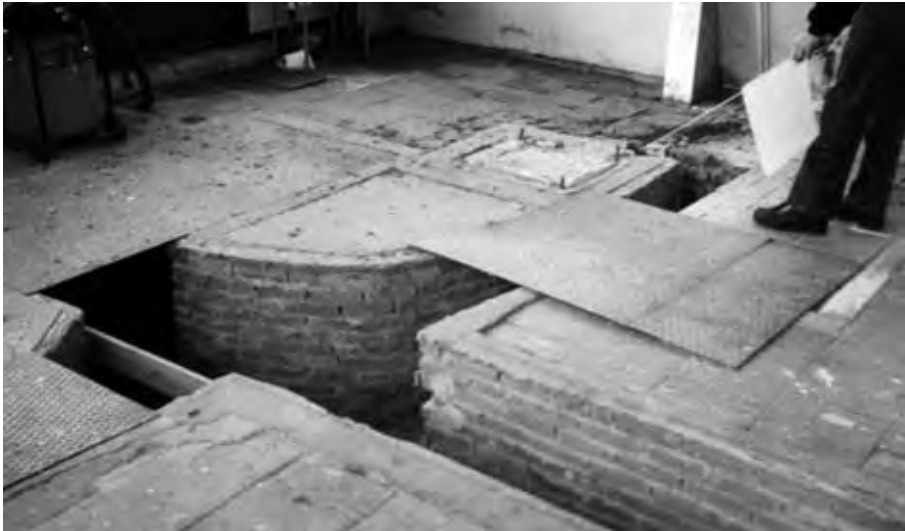
42 Documenting the underground air ducts in the carpentry workshop. They were covered with steel checker plates.
