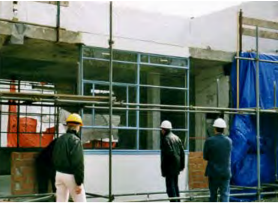
28 In test cases the attempt has always been made to take into account an integral part of the building, as here a part of the façade from the foundation to the roof. The plaster, the finishing of the frames with alkyd paint and the glazing were evaluated.
