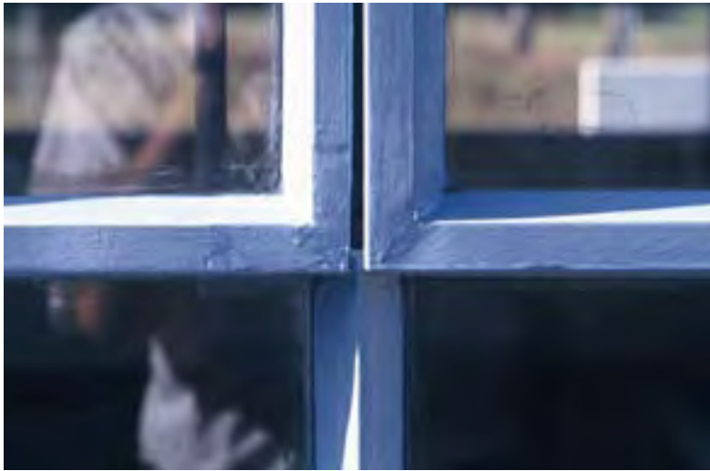
24 Detail of the restored, original façade of 25 mm profile steel. A single T-jamb appears beneath the two adjacent top hung sash windows.
