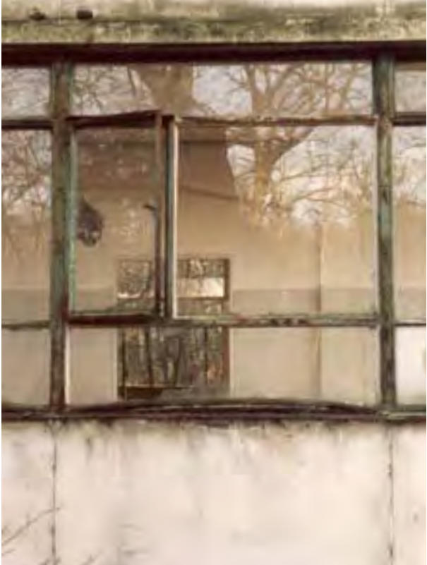
40 A standard window from the corridor walls in the Dresselhuys Pavilion. They were seriously damaged because this side was not protected by a roof overhang. Inadequate profiling meant that the window sills had folded upwards, often leaving the ground sills wet. The consequences can be seen from the swollen steel work of the sills.
