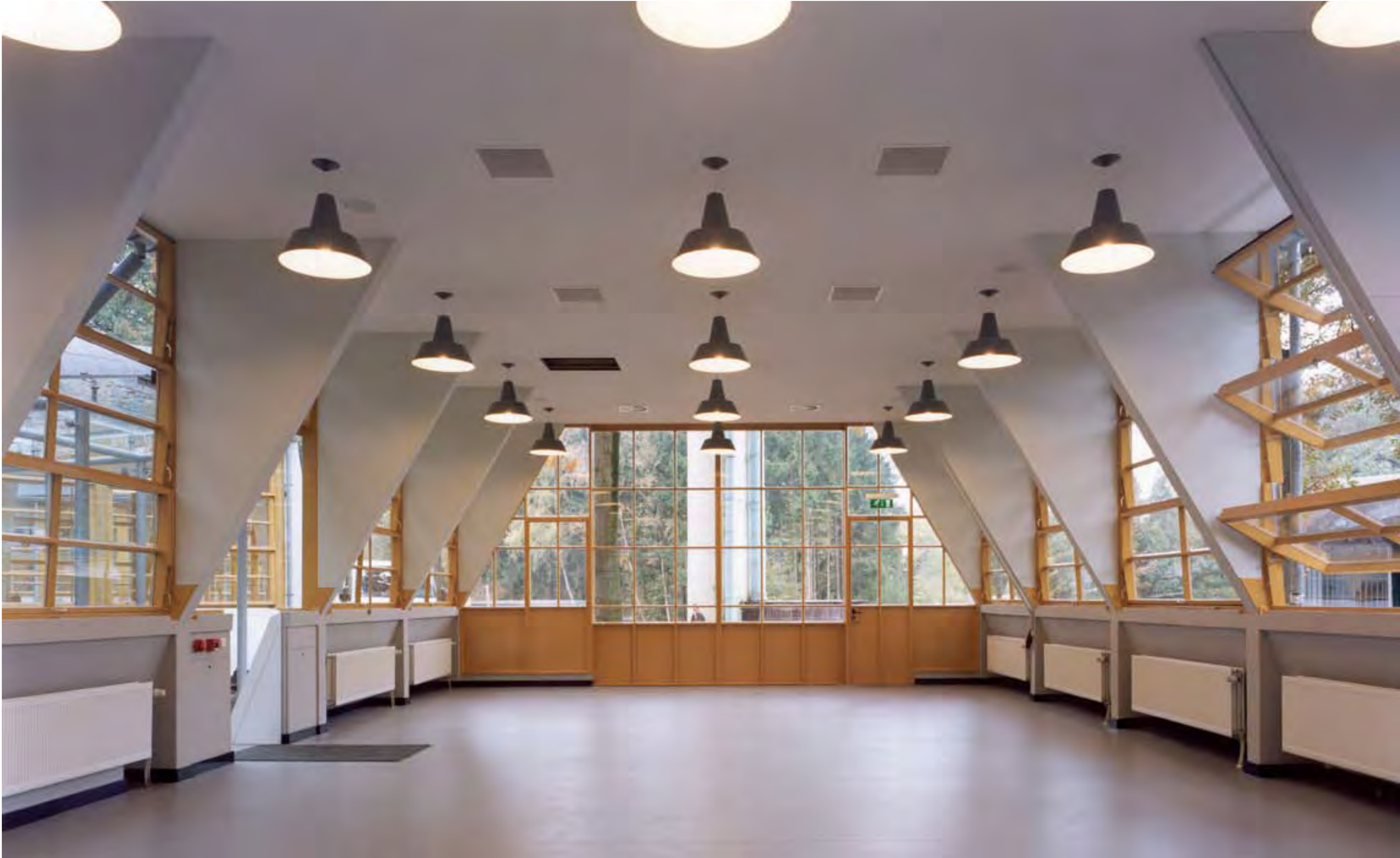
44 The central workshop after restoration. The light fittings are copies, as in the main building, and fitted with PL lamps in a warm light colour.
