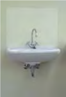
36 Concrete enamel water-proof finish for the walls, which has been meticulously restored. Because the substrate is also different for today's wall plaster, careful planning was required.
