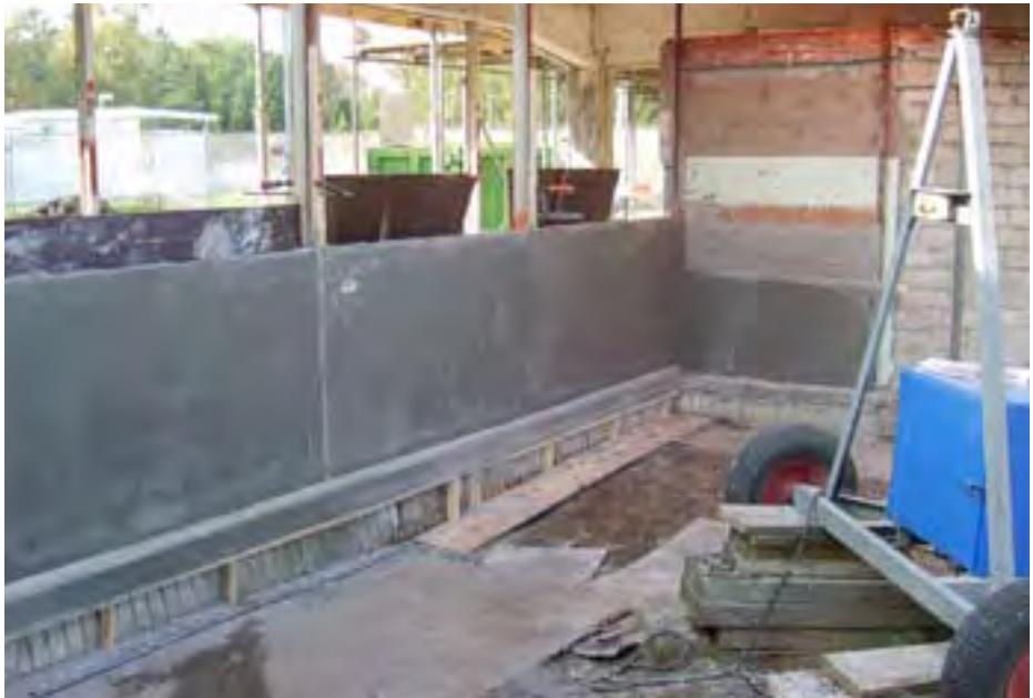
41 The new structure of the parapets. Right the original lime-sand inner cavity leaf. In the middle the new structure with (from inside to outside): cement rendering coat, cavity, thin insulation panel, galvanized steel reinforcement (not visible), stainless steel clayed wire mesh and cement plaster. Left the final result.
