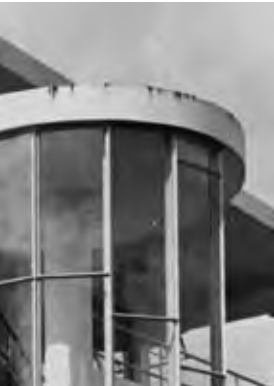
32 South wall of the main building, edge of the roof of the staircase with drip stains from melted roofing tar, 1930s.
