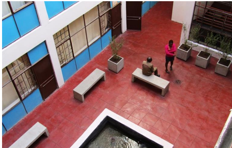
Cooke & Stewart, Aiton Court, Johannesburg, South Africa, 1936-1937. Mayat Hart Architects, restoration, 2012-2014. Central courtyard and water feature viewed from above. © Mayat Hart Architects, 2014.
